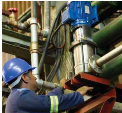
Rowan Moses involved in installing booster pump
